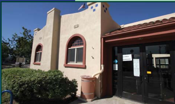
Rain barrel collection system at a branch of the San Diego Public Library
