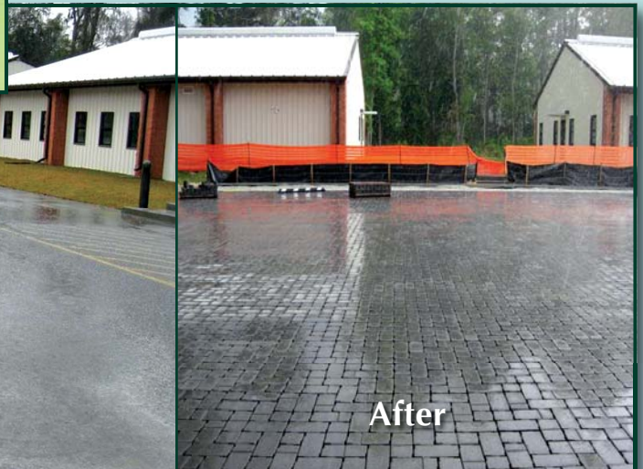
Fort Stewart LID Porous Pavement Project
