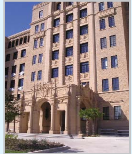
WESTON led the redevelopment of the historic former BAMC hospital at Fort Sam Houston.
