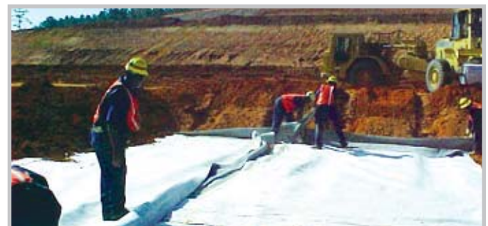
A geo-synthetic clay liner eliminated long-term groundwater monitoring requirements.
